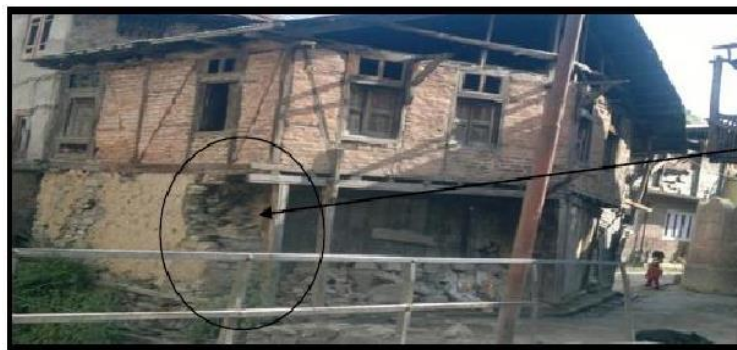
Stage III of Earthquake. Damage
