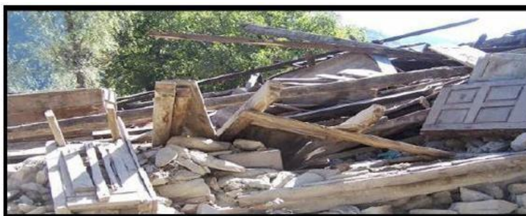
Stage IV of Earthquake. Damage
