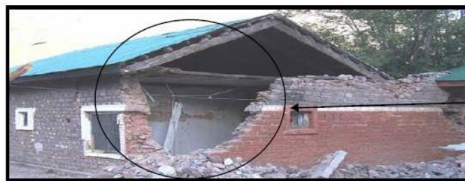
Stage III of Earthquake. Damage
