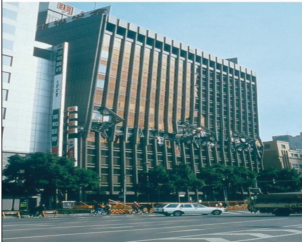
Soft Storey Failure
