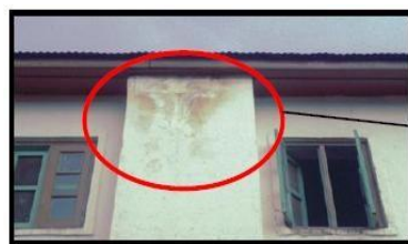
Stage I of Earthquake. Damage
