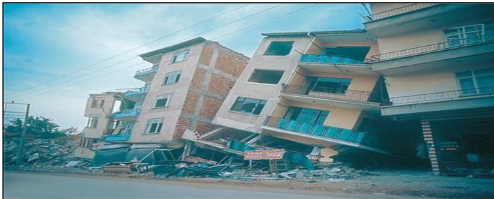
Sway mechanisms are often inevitable with soft storey ground floors (Izmit, Turkey 1999)
